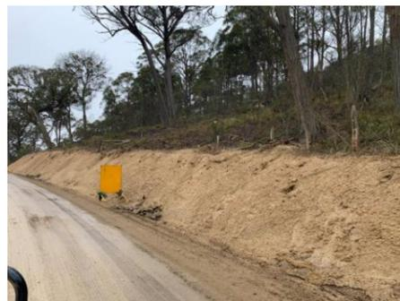
The straw coloured material applied to steeper roadside batters is called Enviro Straw which is an Australian produced hydromulch product. This blend includes a calcium and fertilizer product hydraulic growth medium and Bonded Fibre Matrix. The straw product is thermally treated to remove any weeds, seeds or pathogens during its production.
